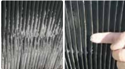
Cooling tower grid
