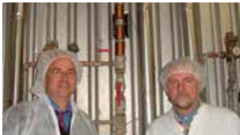
Vulcan installed in a food factory
