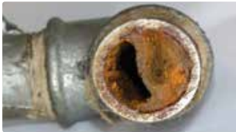
Pipe with scale deposits
